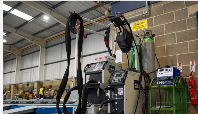
In House Tooling
